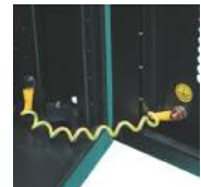
Main parts with earthing knits can connect with each other
